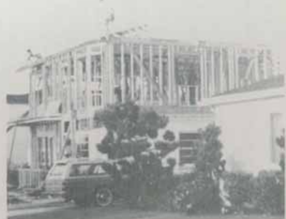
Construction of Second Story Addition
