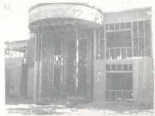
Construction of Single Housing Project
